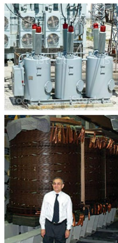
Electric utility substation transformers: outside look, and inside
